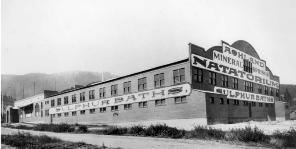
FIGURE 1-13 ■ Ashland, Oregon, mineral springs natatorium. In 1908, local entrepreneurs constructed a large facility over two hot sulfur springs that contained a large covered pool with 58 dressing rooms, balconies around the pool that could seat 500 people, and a ballroom that doubled as an ice skating rink in the winter. (Photo courtesy of the Southern Oregon Historical Society, Medford, Oregon.)
