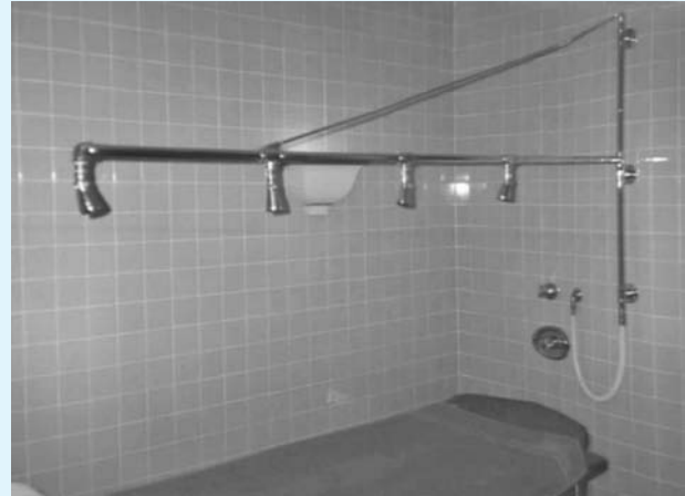
Vichy shower. (Photo courtesy of HEAT SpaKur Therapy Development Inc., Calistoga, California.)
